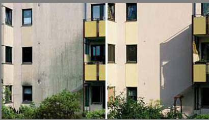
Left: Exterior wall without vs. with STO Lotusan paint
